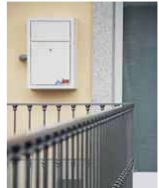
Exhaust air conveyed through special pipeline
