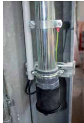
Antistatic vacuum inlet with ground connection
